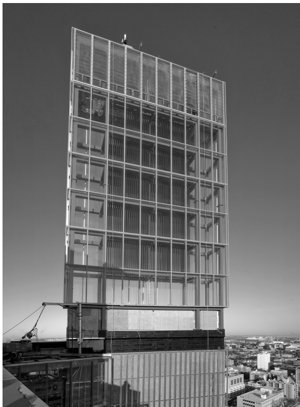
Figure 9: Solar Chimney, Detail, under construction.
